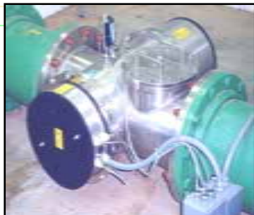
Medium Pressure UV Unit with Flow Sensor Switch
