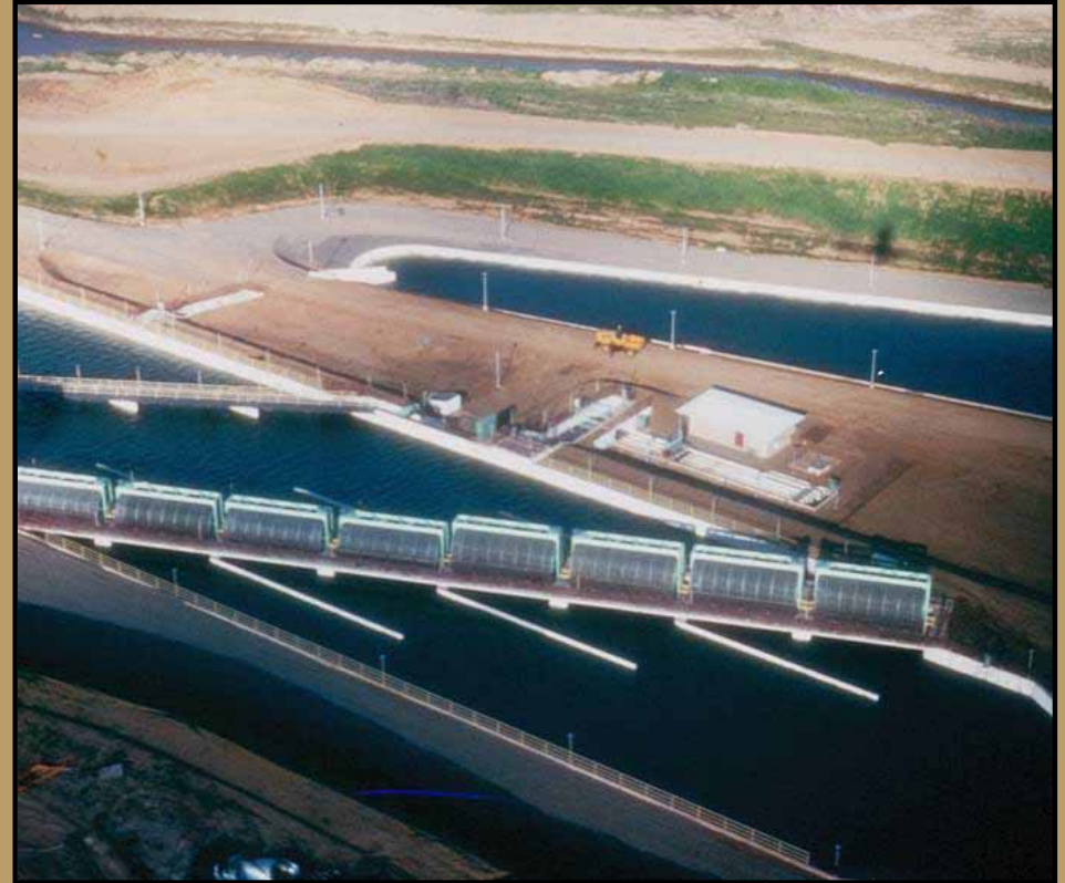
Fish Protection Facilities, PNR
