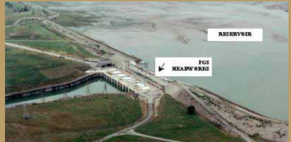
Pump Generating Station
