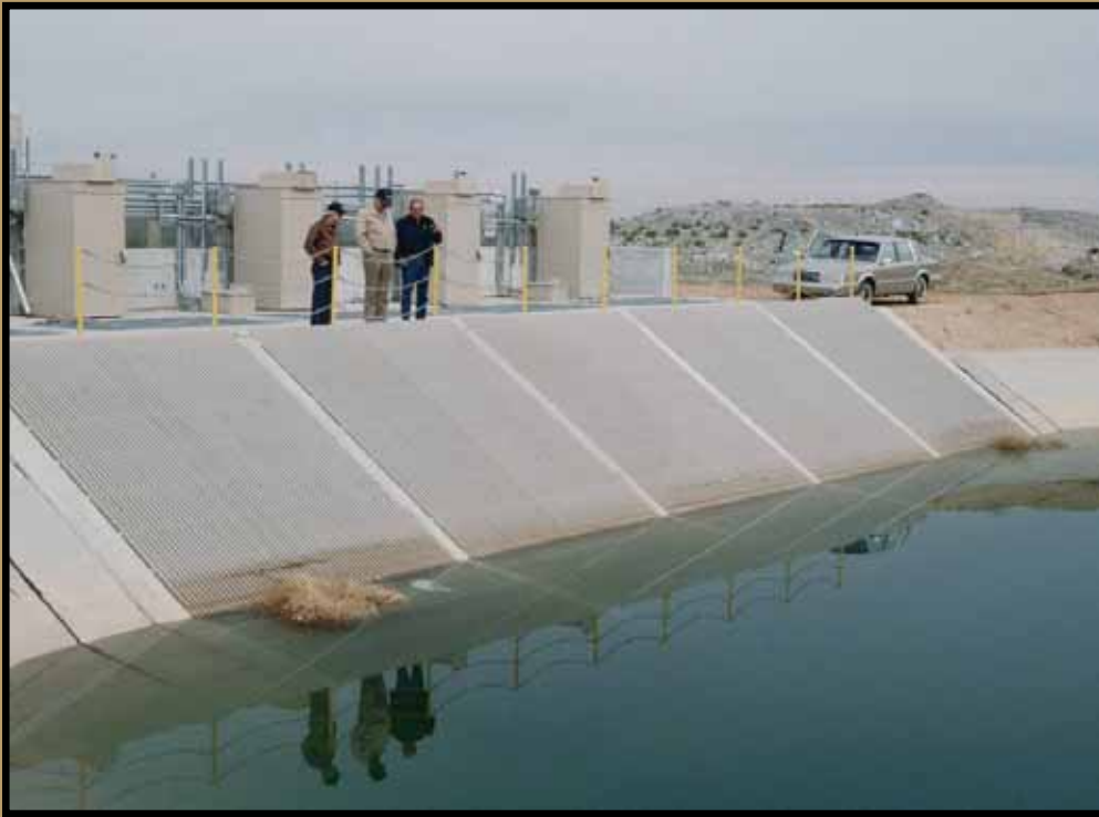
Turnouts and Trash racks
