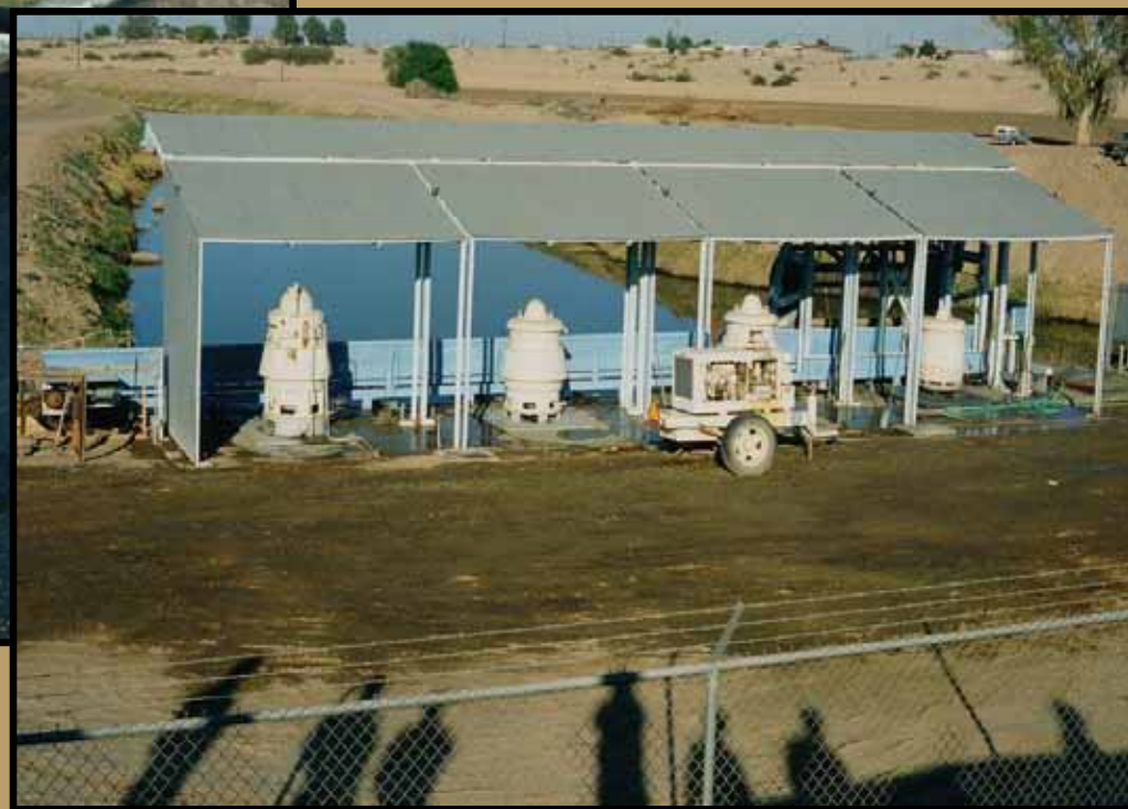
Drain, Yuma Valley Irrigation District
