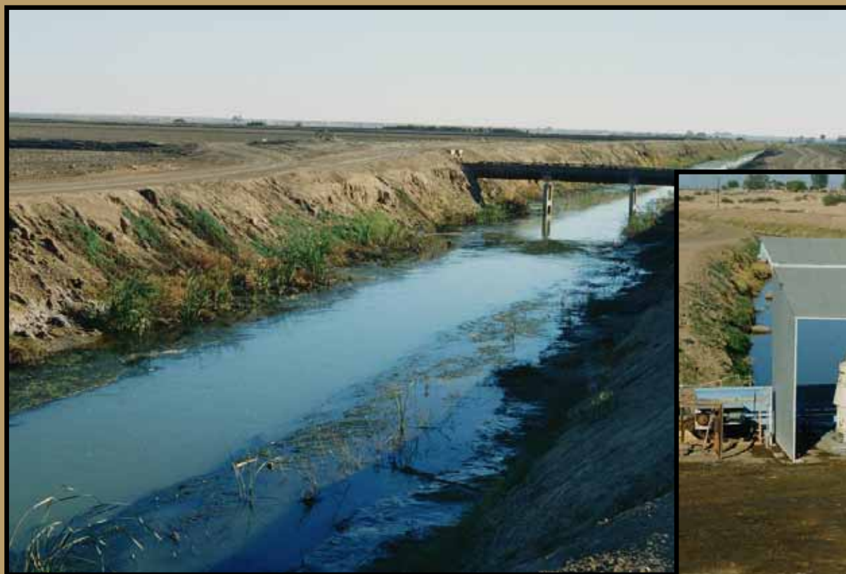
Main Drain, Palo Verde Irrigation District
