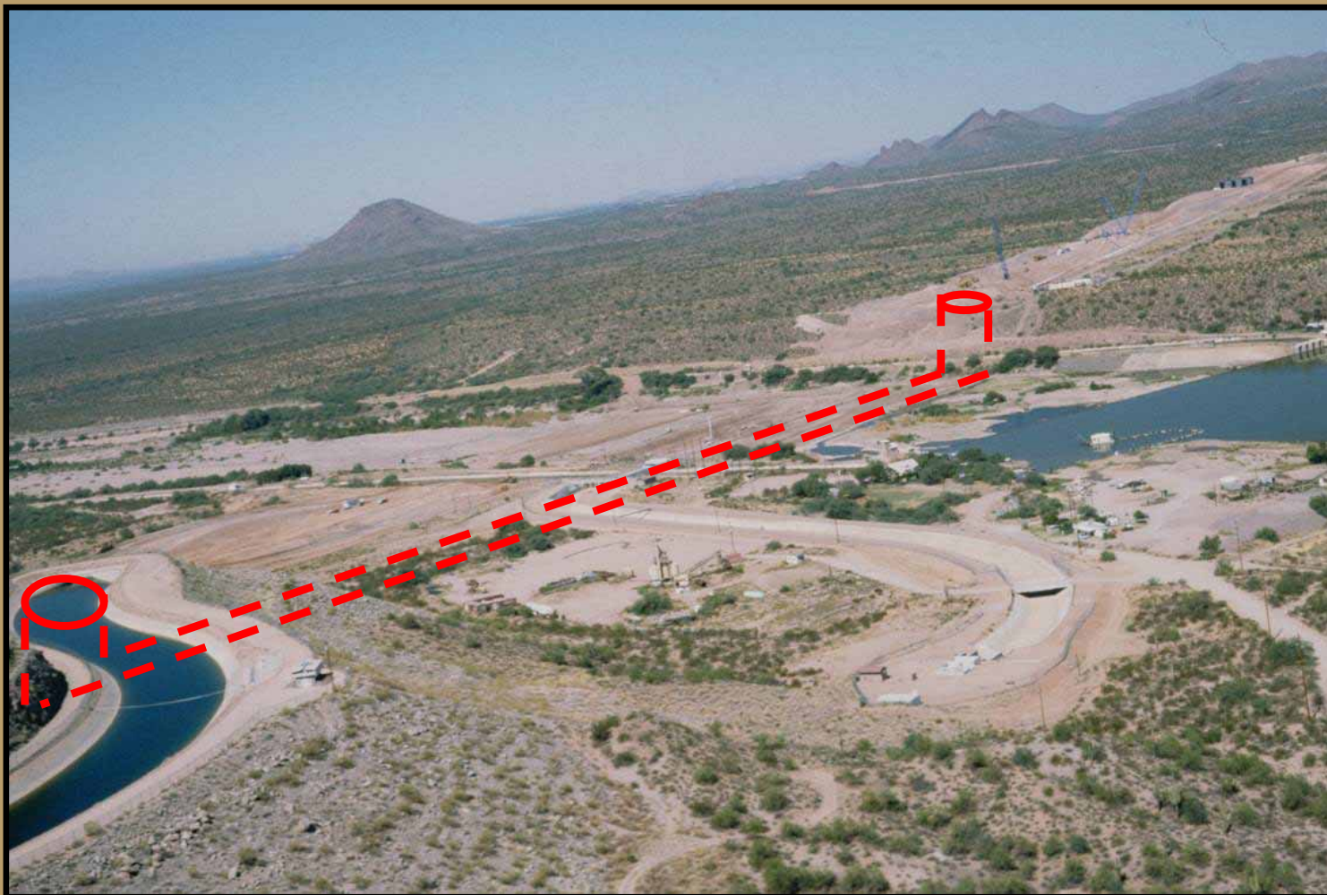
Inverted Siphons – Salt River Siphon (CAP)
