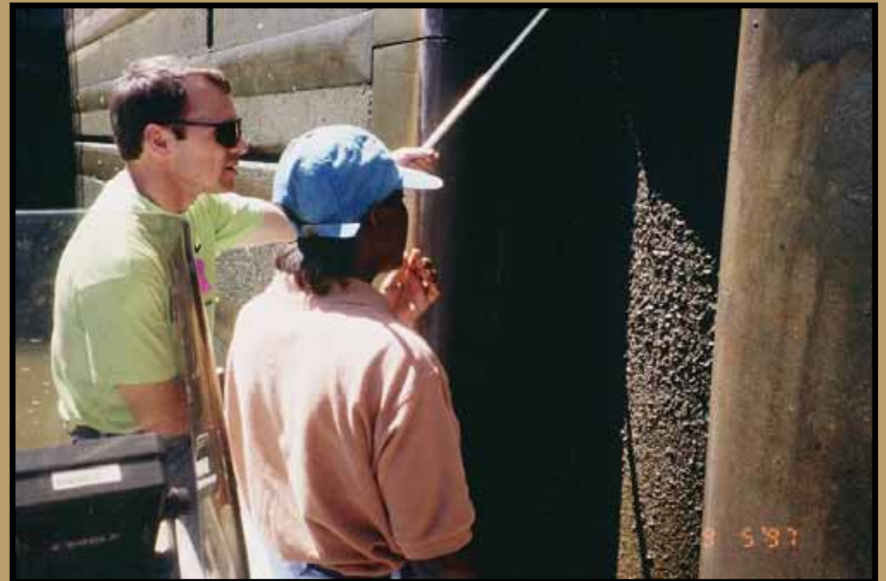
Kerr Lock and Dam (COE), Tulsa OK
