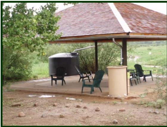
Rainwater barrel & tank at San Pedro House
