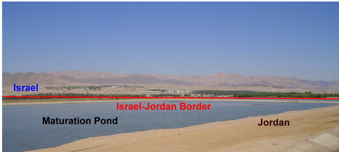
Figure 1. One of the ponds at Aqaba WWTP.
