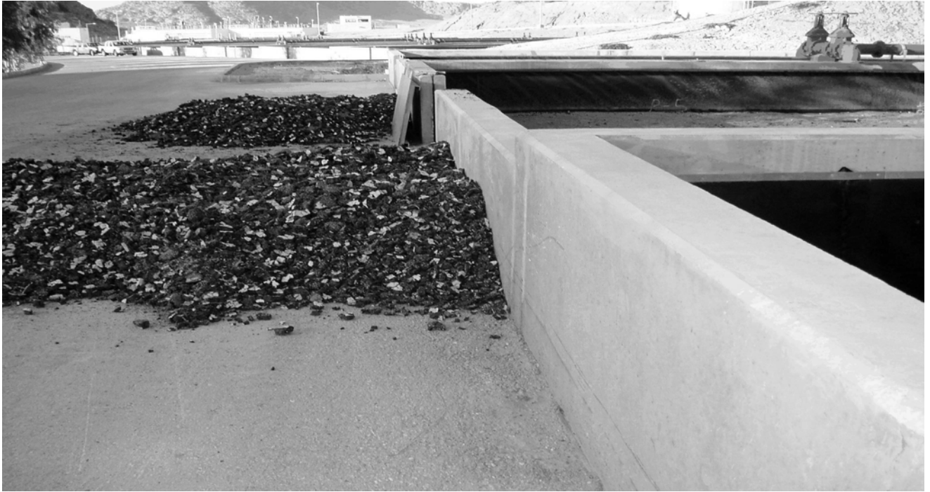
Figure 3. Recent bio-solids in drying beds at Wadi Mousa WWTP-January 7, 2003
