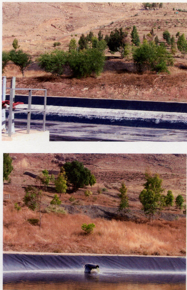
Figure (10): Accumulated disposed sludge at Wadi Al-seir treatment plant.
