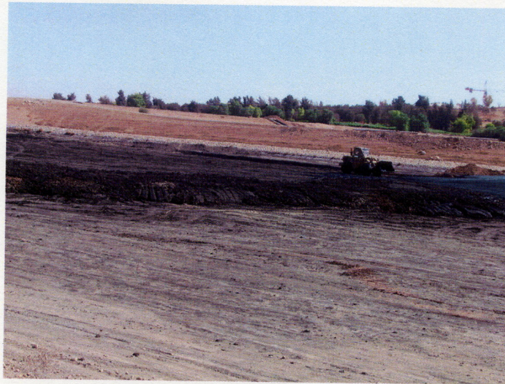
Figure (13): Disposal of sludge at As-Samra treatment plant.
