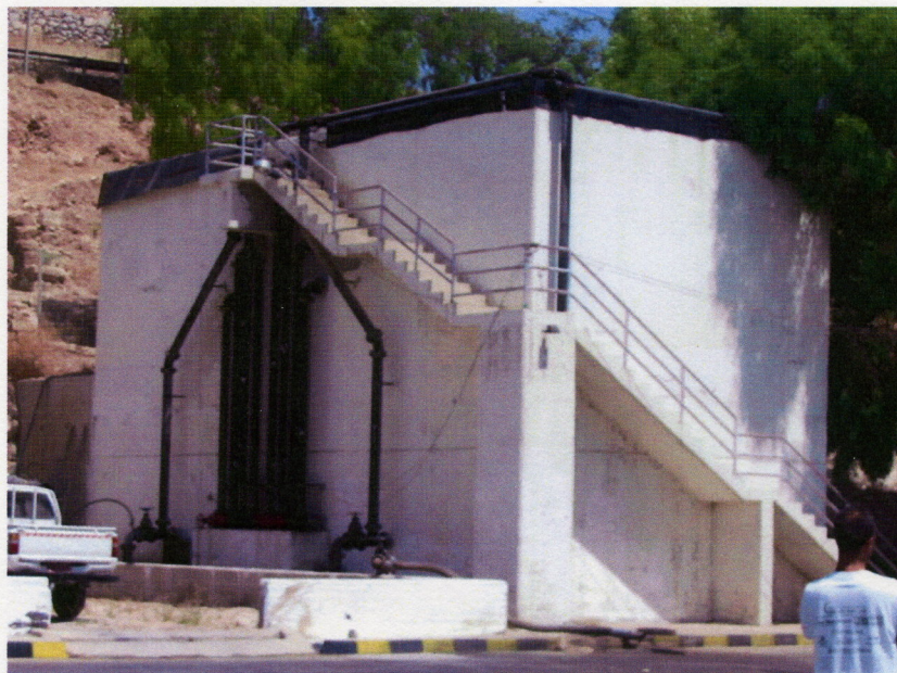
Figure (7): Sludge thickener at Salt treatment plant
