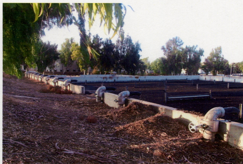
Figure (18): Drying beds at Central Irbid treatment plant.
