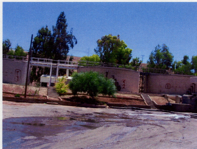
Figure(8): Sludge thickeners at Baq'a wastewater treatment plant.
