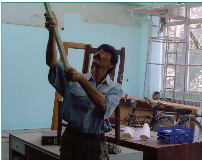
Paint was purchased and painters hired to renovate the room.
