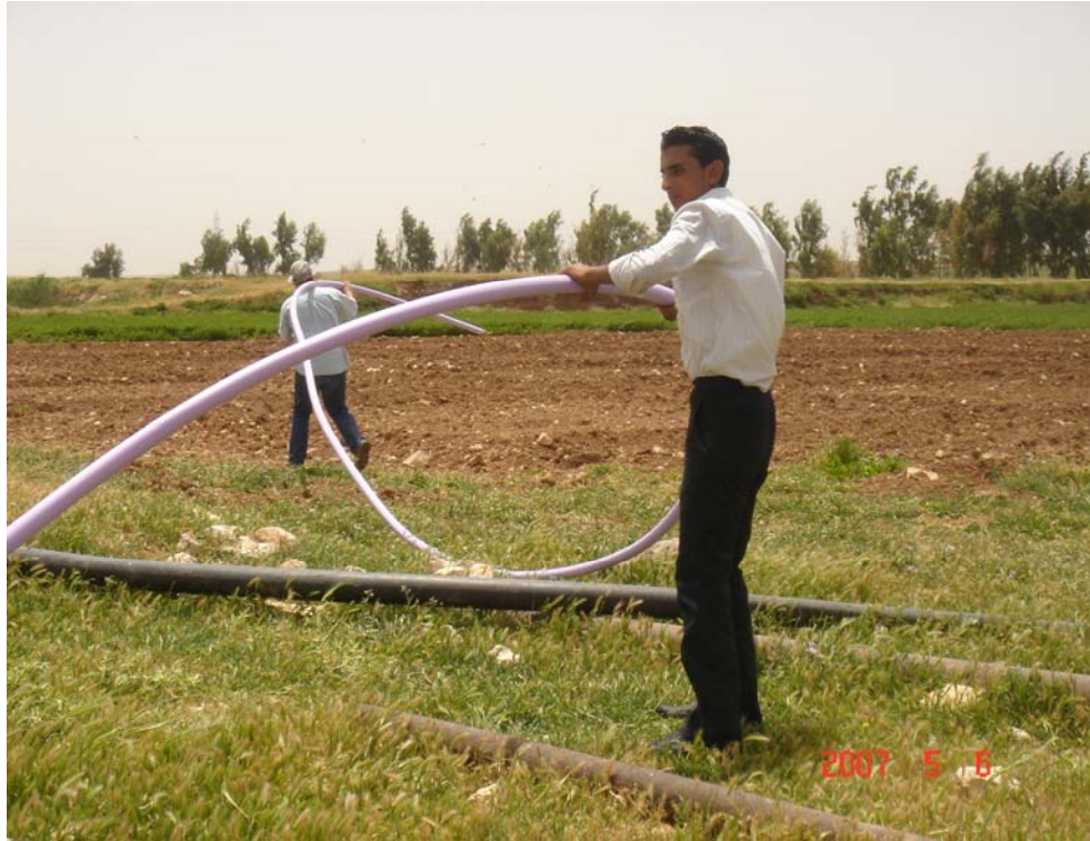
P3: Irrigation system installation
