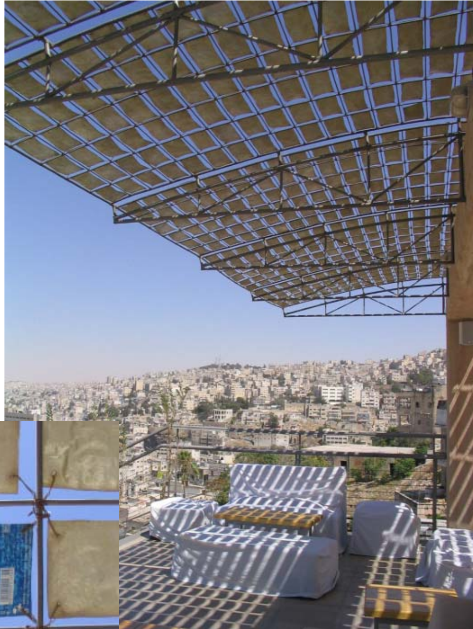
The creative use of discarded soda cans in the construction of a ramada structure at the RSCN Nature Center in Amman by Jordanian architect Ammar Khammash.
