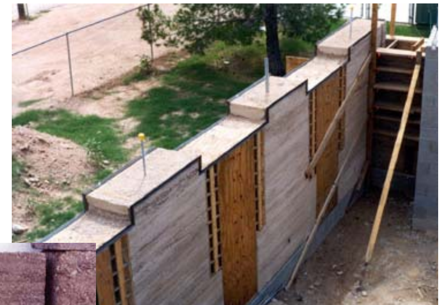
A rammed earth wall being constructed by University of Arizona architecture students - Tucson, Arizona.
