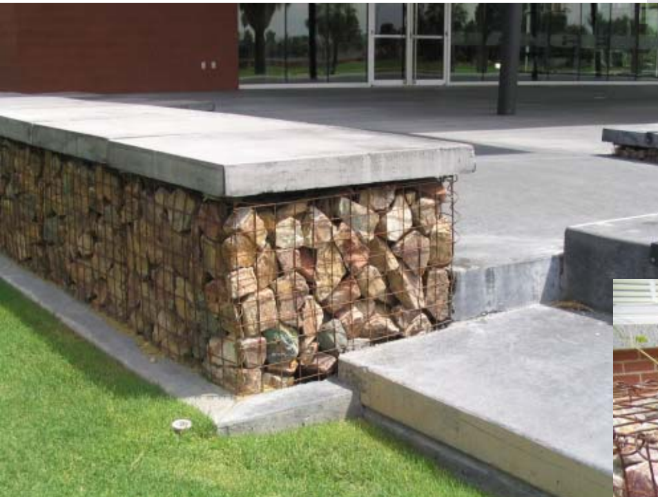
A gabion with a concrete cap creates an attractive seating element at the University of Arizona in Tucson.
