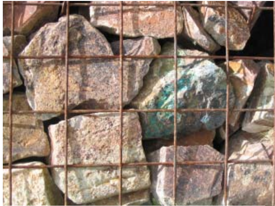
A detail of the rock material creating gabion structures.
