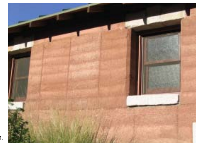
A rammed earth wall being constructed by University of Arizona architecture students - Tucson, Arizona.
