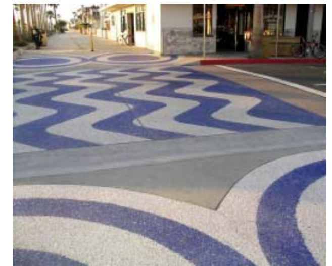
Two views of embedded glass along a pedestrian boardwalk in Santa Monica, California.
