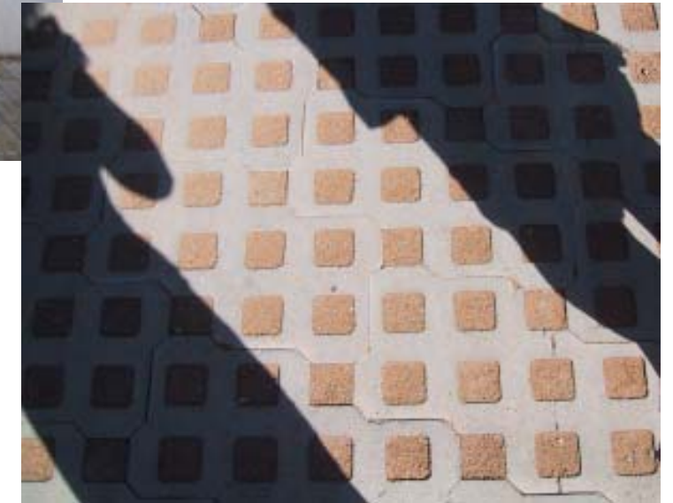
Permeable pavers with stabilized soil in a parking lot - Phoenix, Arizona.
