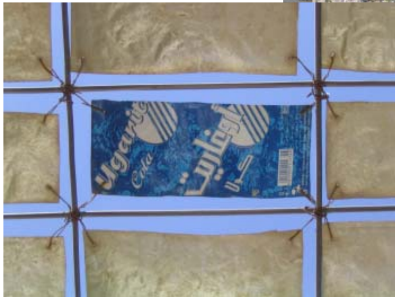
The creative use of discarded soda cans in the construction of a ramada structure at the RSCN Nature Center in Amman by Jordanian architect Ammar Khammash.
