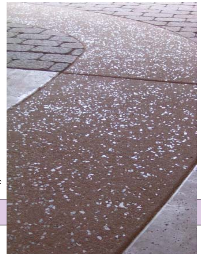
Permeable pavers with stabilized soil in a parking lot - Phoenix, Arizona.
