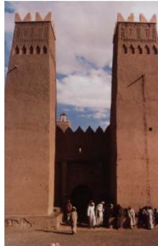
A historic rammed earth structure in Morocco.
