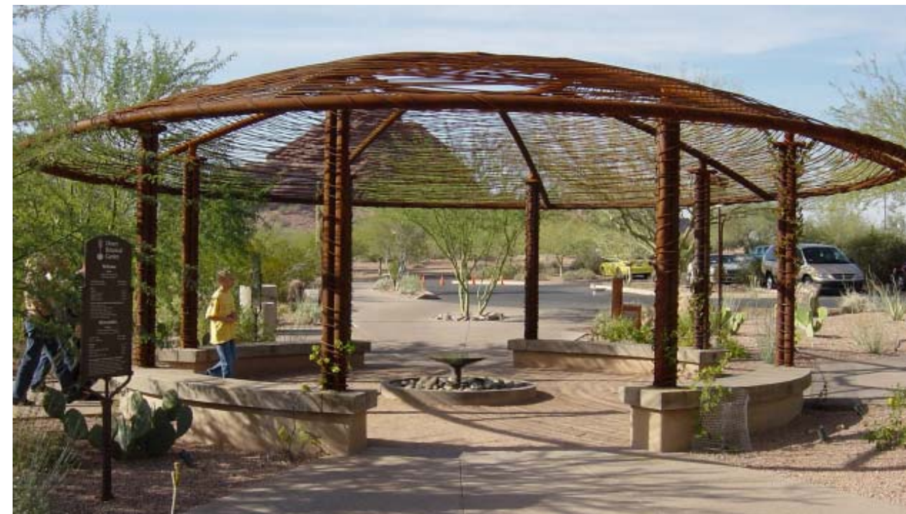
A durable steel ramada structure appropriate for the desert environment.
