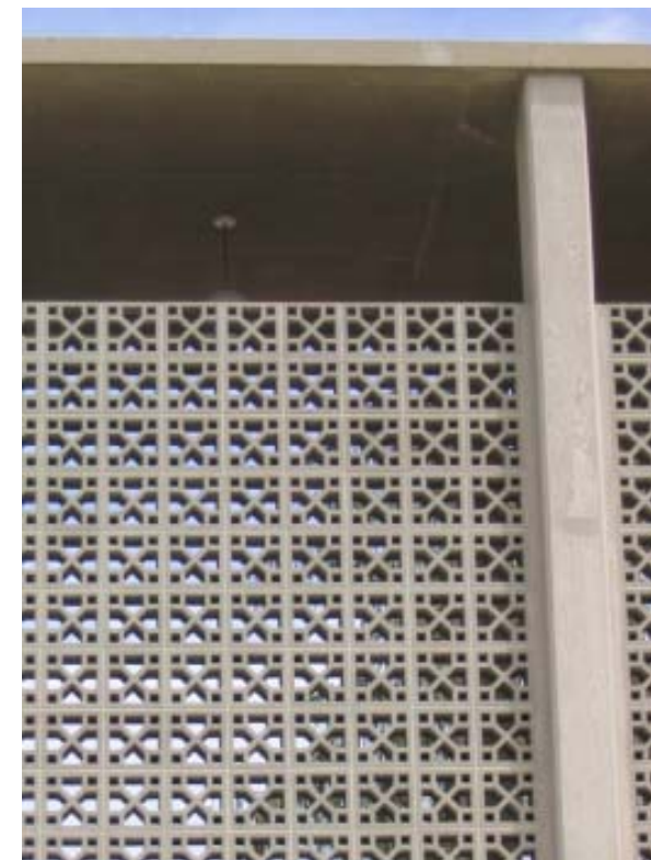
A wall of concrete lattice pieces creates a semi-transparent screen.
