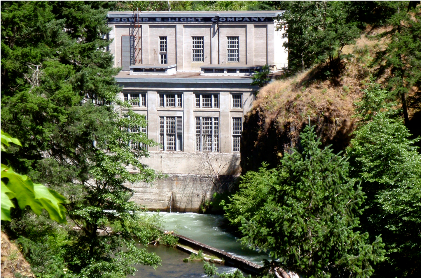
FIGURE 1 - Dam Site before removal
