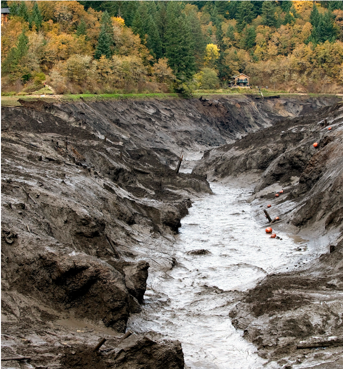
FIGURE 5 - Post-dam removal flow through Northwestern Lake (White Salmon River (c)www.columbian.com, CC BY-NC-SA 2.0)
