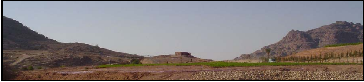
Figure 10: the existing structure on location of proposed interpretive center
